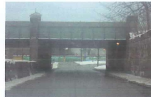
Fig. 10- Inactive Rail Viaduct crossing over Amherst Street
