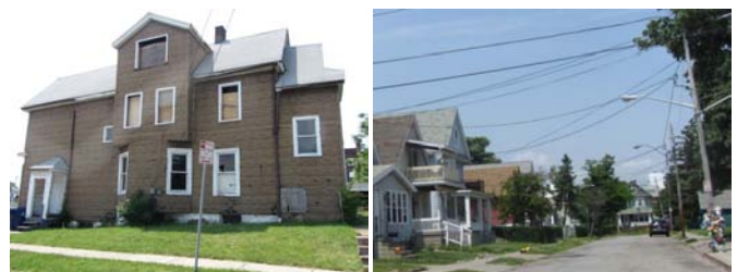
Figures 23 and 24: On left, a house remains boarded up after a fire. On right, a streetside memorial tied to a pole catches the eye amidst unkempt lawns. Takeaway: Visual blight should not endure and spread.
